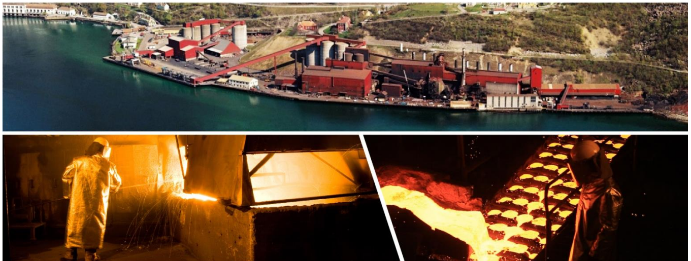
TiZir Titanium & Iron ilmenite upgrading facility, Tyssedal, Norway
