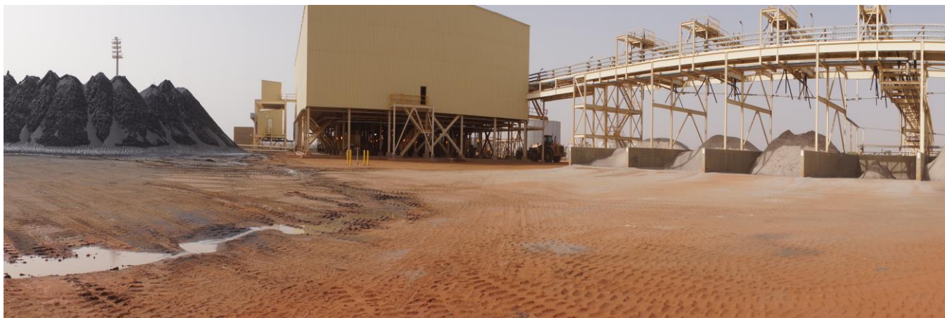
Grande Côte Mineral Separation Plant
