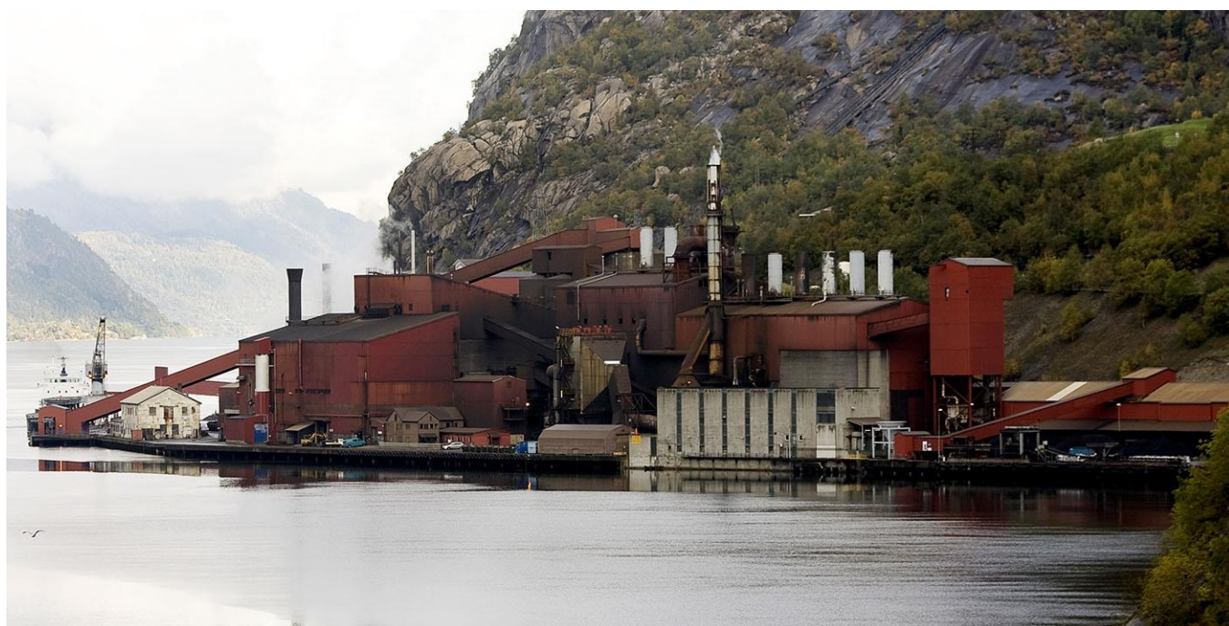
Tizir Titanium & Iron ilmenite upgrading facility, Norway
